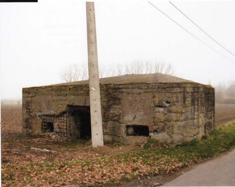
▲ Bunker A6 (foto Bunkergordel)
